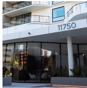
LANDMARK TOWER II
