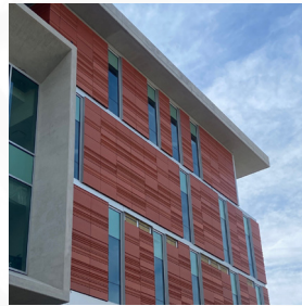
UNLV MEDICAL EDUCATION BUILDING WWCCA Project of the Year
