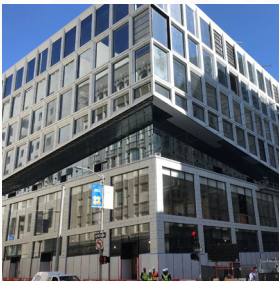
120 STOCKTON WACA Construction Excellence
