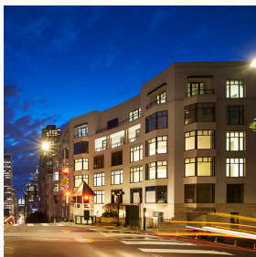
875 CALIFORNIA AWCI Excellence in Construction Quality
