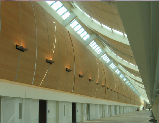
SAN JOSE AIRPORT TERMINAL B
